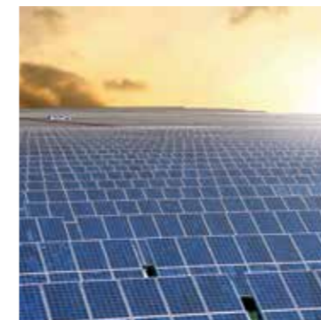
➤ Photovoltaic panel mounts
