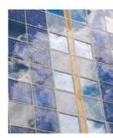
Building integrated photovoltaics (BIPV)
