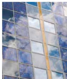
➤ Building integrated photovoltaics (BIPV)
